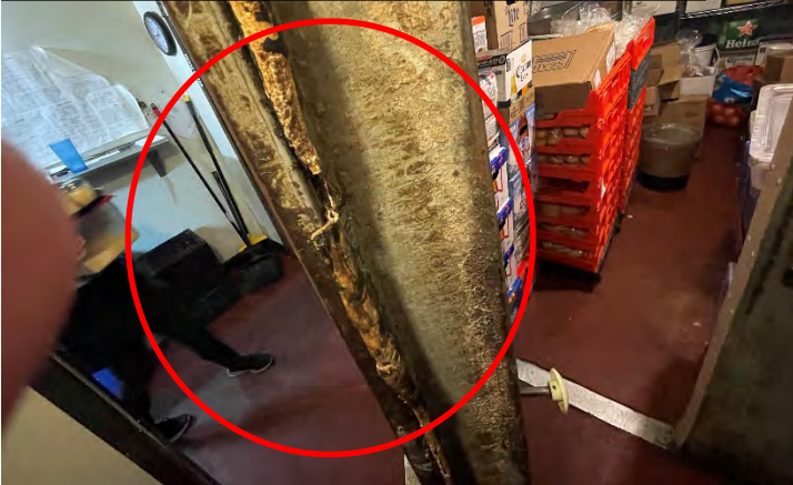
Facility in poor repair – damaged and torn gasket on walk-in cooler door
