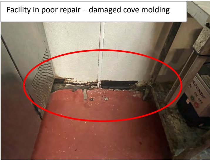
Facility in poor repair – damaged wall
