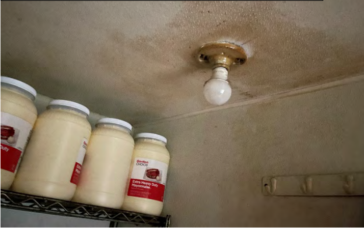
Lights not protected – bulbs not shatterproof or covered with shatterproof covers
