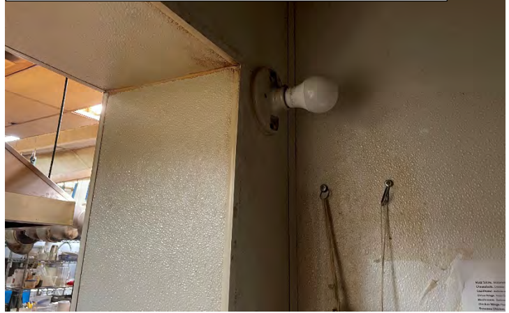
Lights not protected – bulbs not shatterproof or covered with shatterproof covers
