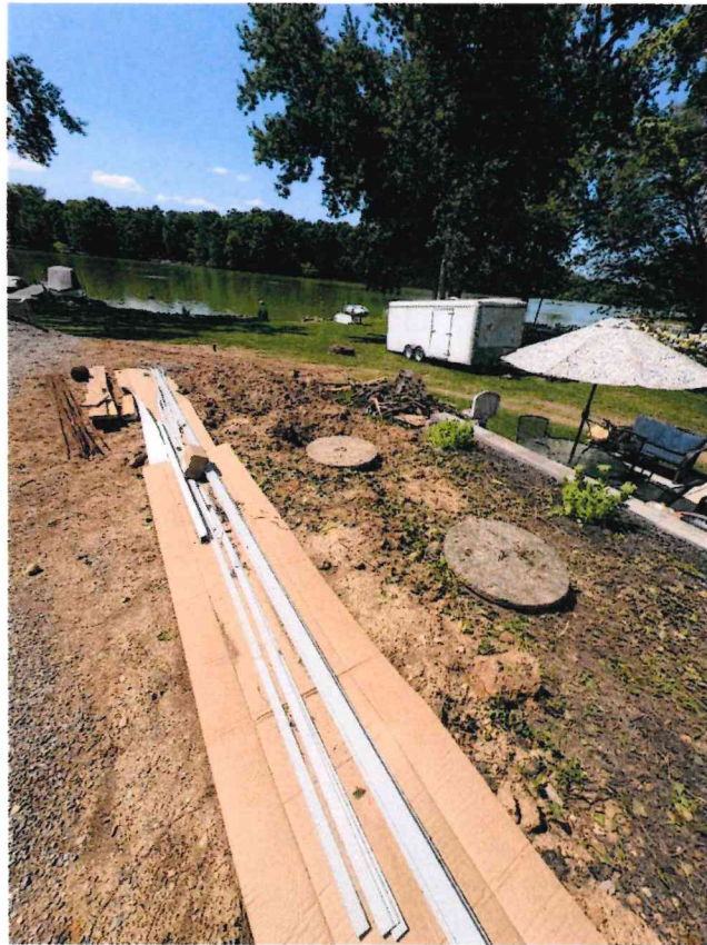
View of edge of disturbed area from edge of pool framing
